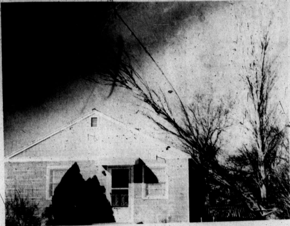
COME ON IN, DON'T BOTHER TO KNOCK — Mr. and Mrs. C.M. Smith of 229 Ave. D. were somewhat surprised when the tree next to their house came crashing down on their roof during the high winds Thursday afternoon. No extensive damage was reported, but their television antenna was bent by the wind.
