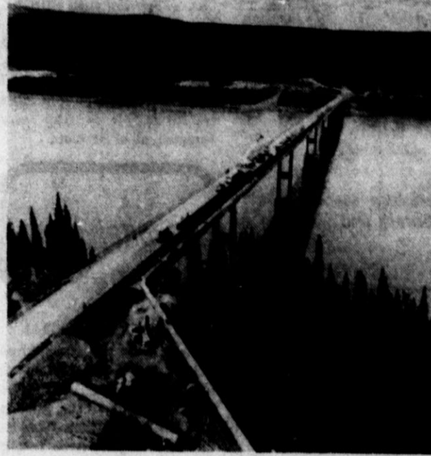
ONE CRITIC SPECULATES that if the 2,300-foot Yukon River bridge were blown, the damage to the Alaska pipeline would reach well beyond the cost of reconstruction.
