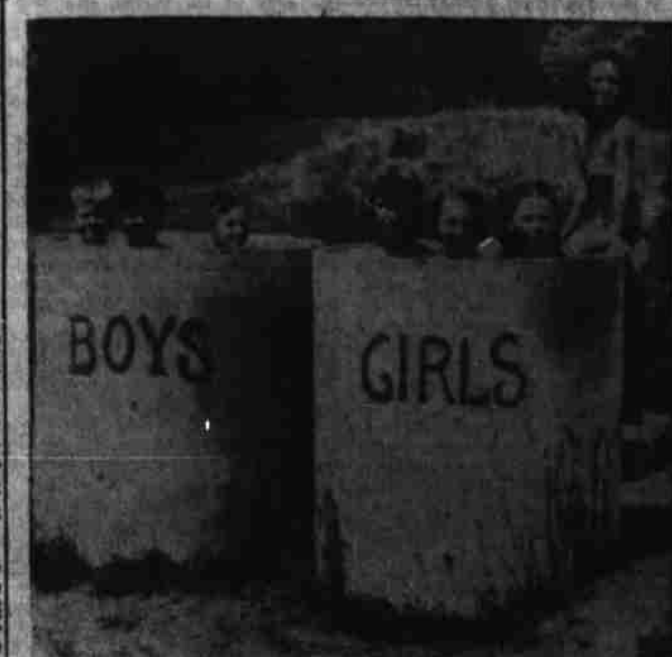
BATHHOUSES — Boys and girls of Lincoln, Vermont, change their clothes in two country-style bath houses installed at the OJ swimming hole by Lincoln residents for the sake of modesty of their young 'uns. They are sections of concrete culvert, up-ended and appropriately labeled. (AP Wirephoto).
