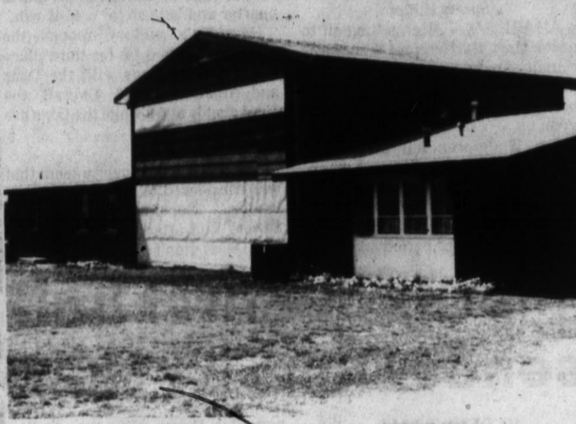
ST. THOMAS EPISCOPAL CHURCH ...building under construction
