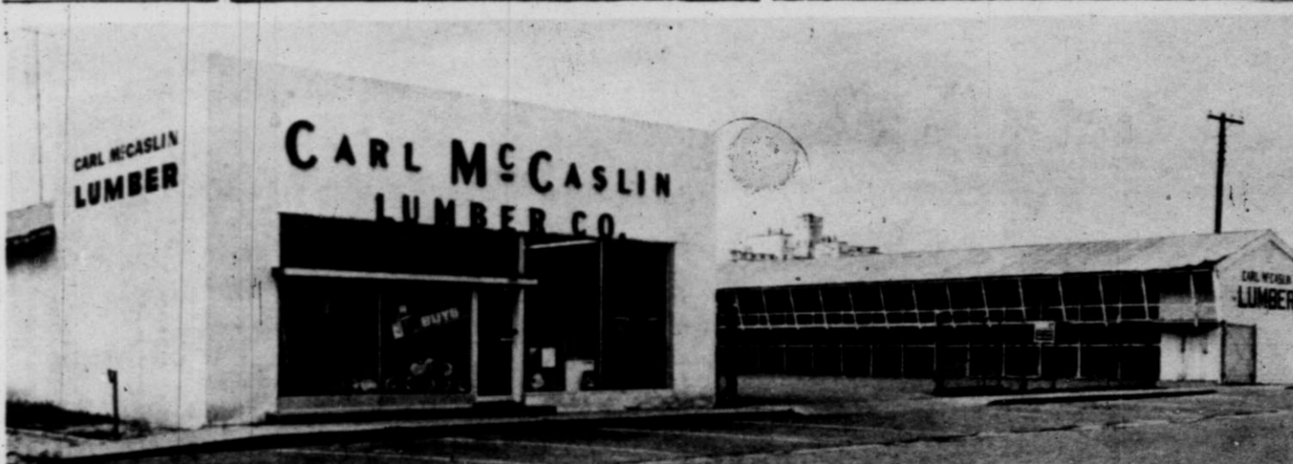
MANY CHANGES have been made since 1939 which has included a number of remodeling programs. The display room has been tripled in size,
