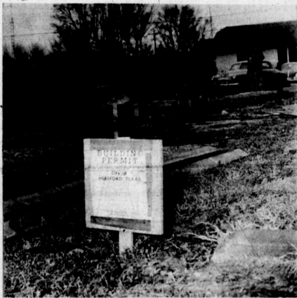
GROUNDWORK on Chamber of Commerce home
