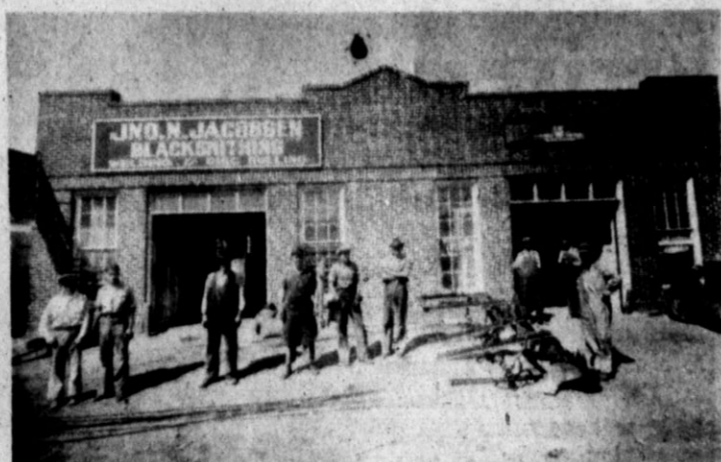
REBUILDING — This new building went up at the same site in 1929. From left, those in the picture are J. W. Cawthon, helper; Berry Jacobsen; John N. Jacobsen Sr.; B. Bandy, helper; Chris Jacobsen; John N. Jacobsen Jr.; and customers Wolf, Harry Teitjen and Fred Winfrey.
