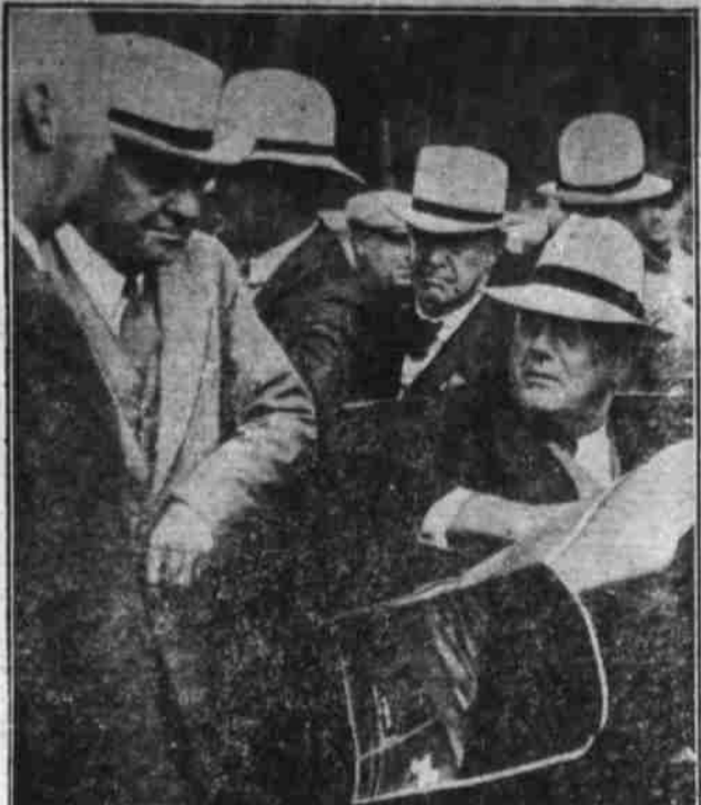
President Roosevelt is shown as he discussed blueprints of the $31,000,000 Bonneville power and navigation dam project, on the Columbia river 40 miles from Portland, Ore., when he visited there on his return trip from Hawaii. At left is Secretary of War Dorn. (Associated Press Photo)
