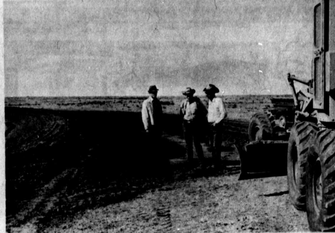
ELIMINATING EROSION — A. C. Hays, left, and Tom Hargrave and Buster Sublett look over the work being done on Hays' ranch land that is expected to help in curtailing the
