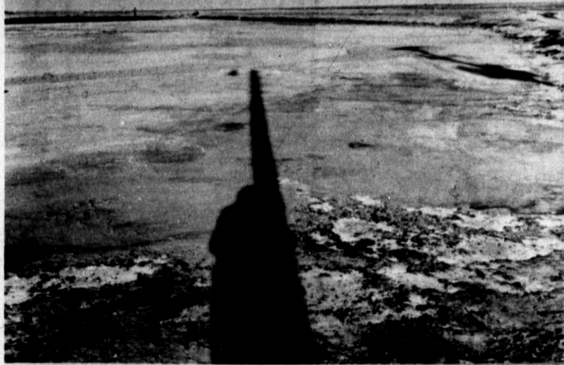
FILM OF SALT — Just a glance at an area of land southeast of Hereford produces a likeness to the barren moon surface. Evaporating basins at the Hereford Salt plant, which many persons are unaware exists, extend over several acres with low dikes separating the pools where the brine dries and leaves a film of salt. —Photo by Sue Coleman
