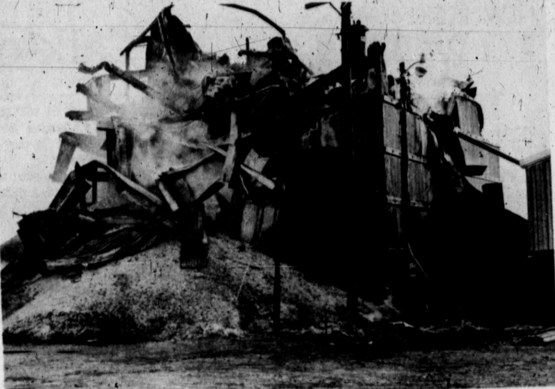
COSTLY FIRE — This private Grain elevator located about 20 miles north of Hereford, suffered an estimated $170,000 in losses from a fire which occurred early Thursday morning. Local firemen fought the blaze for about six hours before getting it under control.
