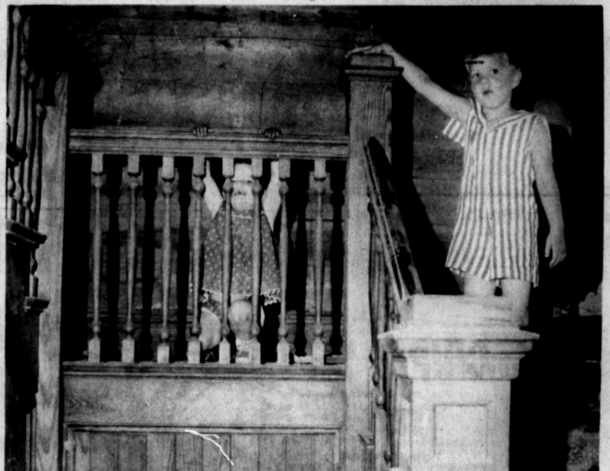
STAIRWAY POST is measured by Diana Devers with a serious air, although her little sister Monica clowns as she peeps through the railings on the landing. The handsome, solid
