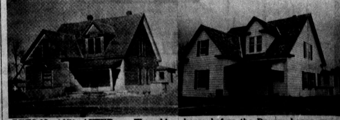
BEFORE AND AFTER — The old Jennie Thompson place, at 515 Union, has begun to take on a new look since Bill and Elva Devers began working on it recently. The photos show the house before the Devers began renovating it and how it looks now. Other photos and a story of the Hereford landmark can be seen on Page 6 of this section. —Staff Photos
