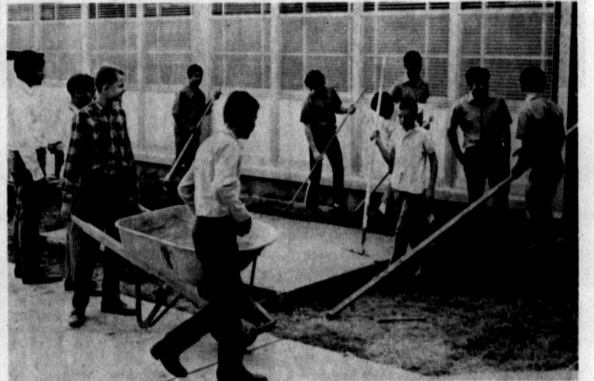
BUILDING TRADE — Students in the La Plata building trades class are shown putting the finishing touches on a concrete foundation at the school which will serve as a base for a small storage building in the school's patio.
