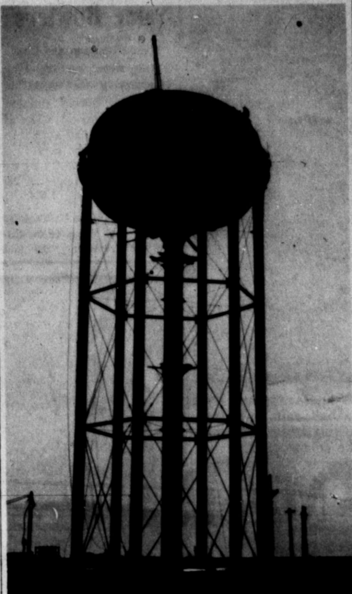
AWESOME GIANT — The size of the giant water tower which is to provide water for the Wilson and Company plant, can be depicted by comparing it to size of the workman near the upper right corner of the dome. The tower will hold an estimated 400,000 gallons of water. —Staff Photo
