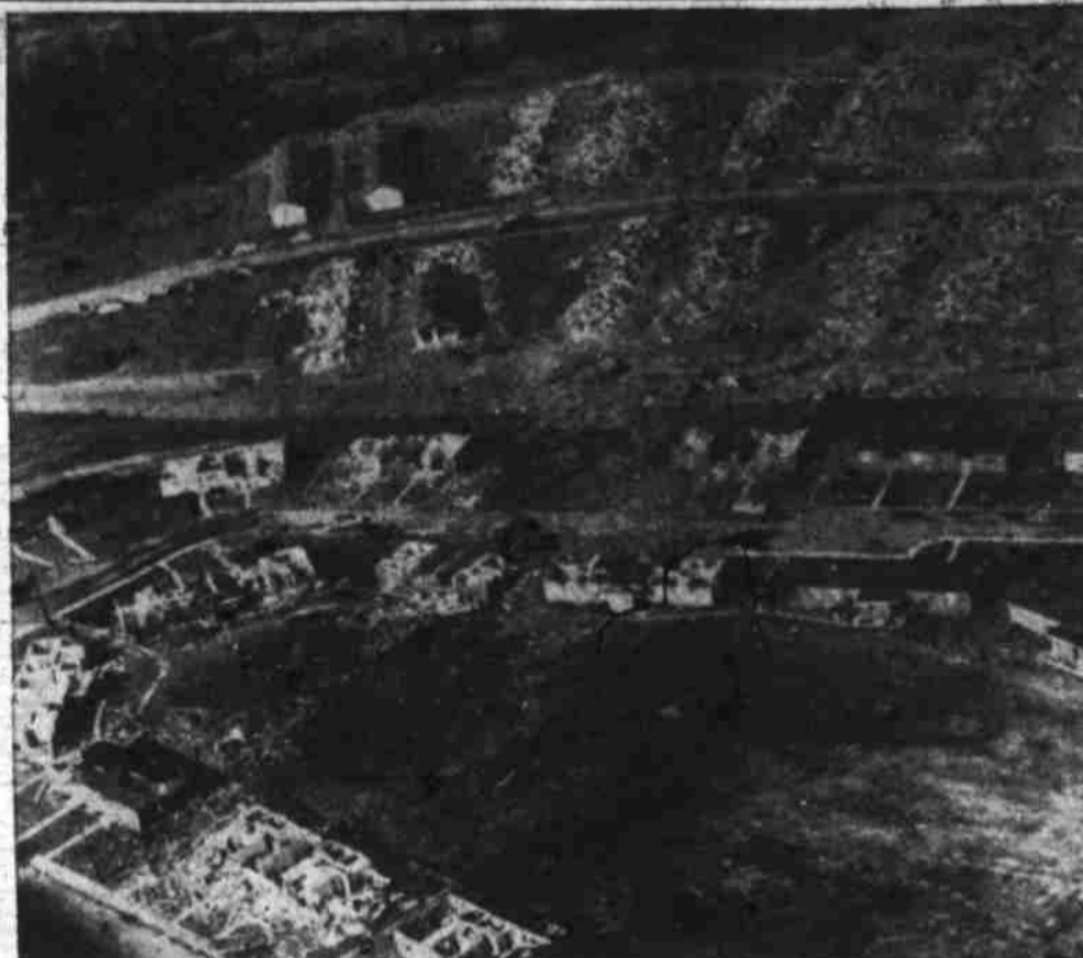
Tornado Damage. This is an air view of the destruction caused at Warner, Ga., by a tornado that struck just before dark Thursday. Fifteen persons were killed and 150 others were injured. Properly damaged was estimated in the millions. (AP Wirephoto).
