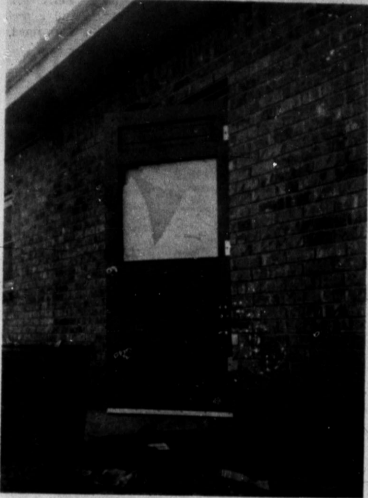
VANDALISM — Last week, vandals broke into the Camp Fire Lodge through the back door, causing damage to the door. Also taken by the vandals were several fire extinguishers, juices and foodstuffs. —Staff Photo
