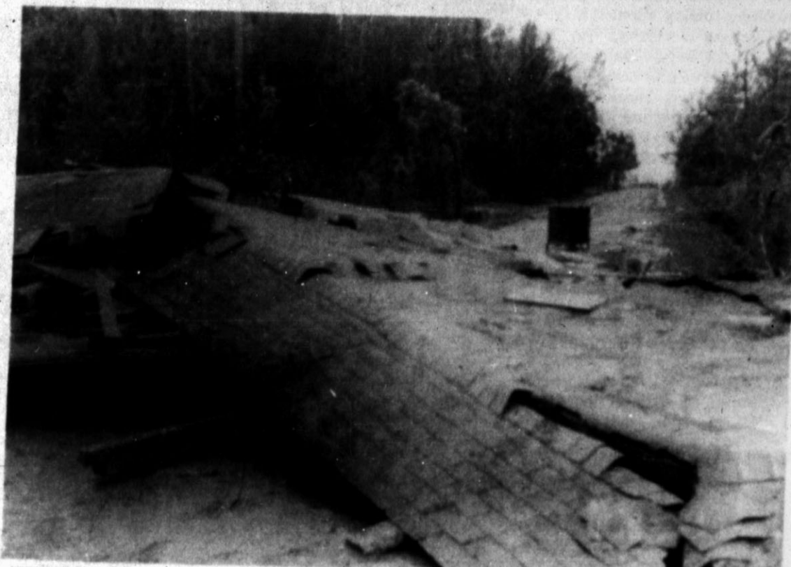
HURRICANE CAMILLE — This scene of devastation, photographed by Clark Andrews of Frío on the spot in Biloxi, Mississippi, last week, gives some indication of the property loss in the Gulf Coast area. Mrs. Andrews' accounting of their experiences in Biloxi offers greater details.
