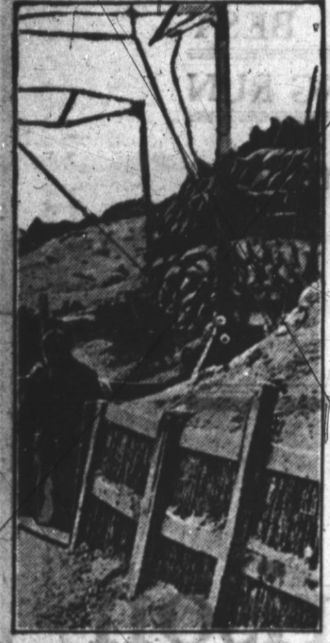
Entrance to a Dugout.
