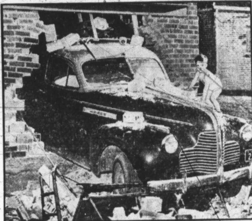
All that Kenny Keenan, 2 1/2 of Pueblo, Colo. did, was to step on the starter of his grandfather's shiny new car, parked in the driveway. The car rolled down the drive, gathered speed, went through the garage and out the rear wall. No one was hurt.
