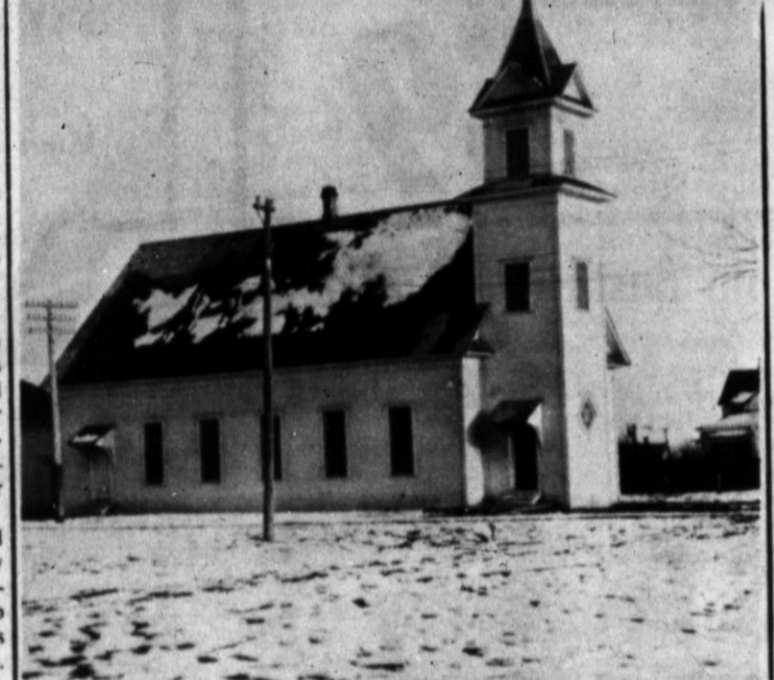
FIRST BAPTIST CHURCH — Gladys Manjeot, publicity chairman for the Mid-Plains Pioneer 1968 Celebration set for May 30 at the Bull Barn, released her own picture of Hereford's first Baptist church, which was constructed during the early 1900's with a bell tower, then located on Jackson and Fourth streets.
