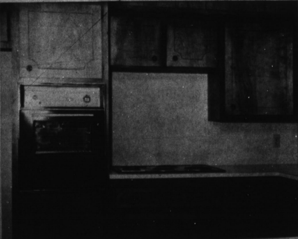
Total Electric Kitchen includes built-in range and oven, dishwasher, food waste disposer and vent hood.
