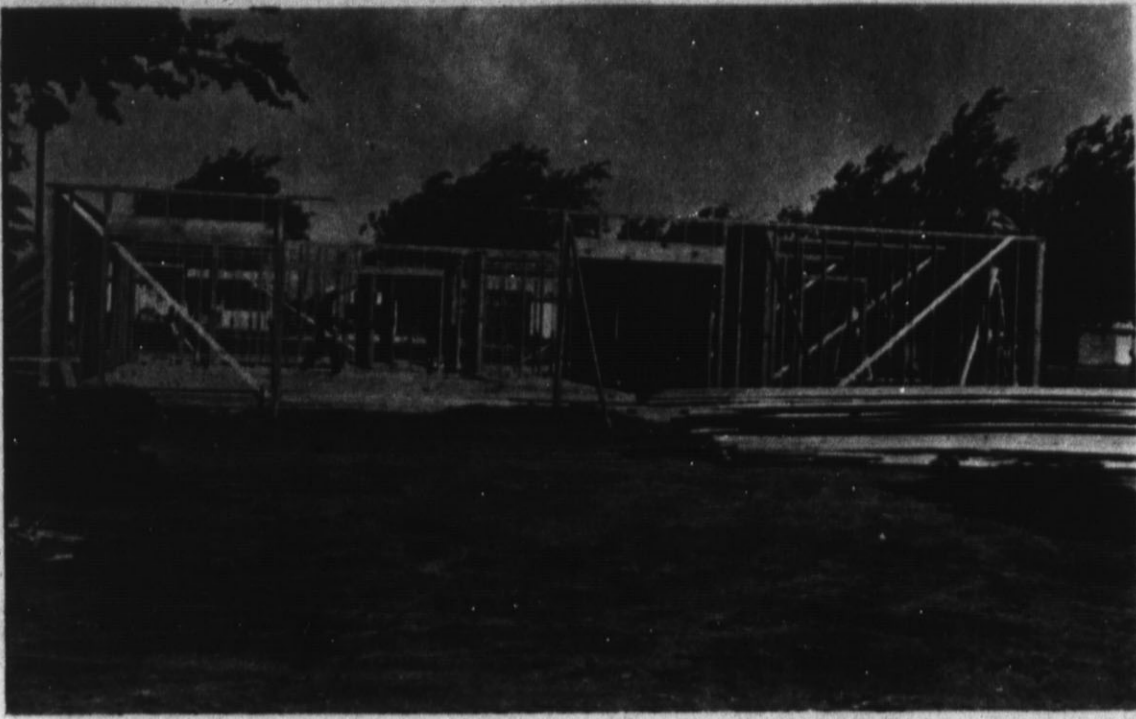
GOING UP — After laying the foundation for the Campfire hut, workmen have now begun constructing the wall for the building. Joint efforts by the Hereford Rotary and Lions Clubs, along with a $13,000 grant from the Jim Hill Estate, are aiding in the construction of the building.
