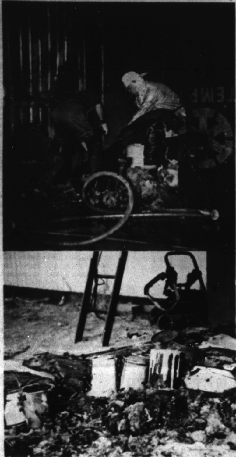
FIRE DAMAGE AND PROBABLE CAUSE —Damage to Allied Millwrights, located west of the city, was estimated at more than $1,000 following a fire there Sunday morning. The blaze, which was contained to office spaces and the walls around that area, was believed to have started when cans of paint near a heater became too hot. Two units of the Hereford Volunteer Fire Department answered the call and remained at the scene about 40 minutes. There also was much smoke damage.
