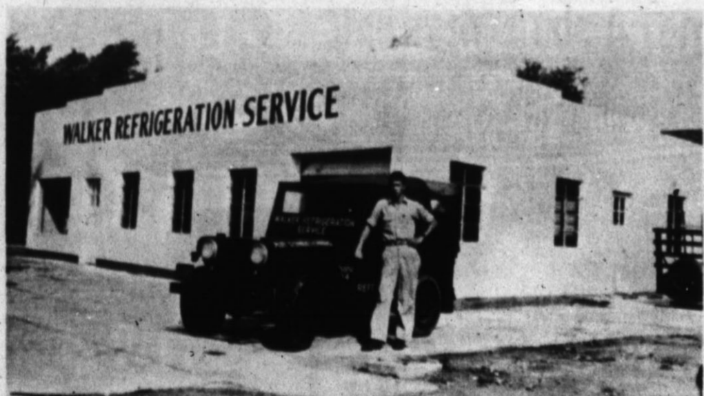
SECOND LOCATION — Walker Refrigeration Service moved to its present location in 1947 and an employee of Walker's then, J. D. Paorch, is shown with the newly remodeled building. (Photo courtesy of Dick Walker)
