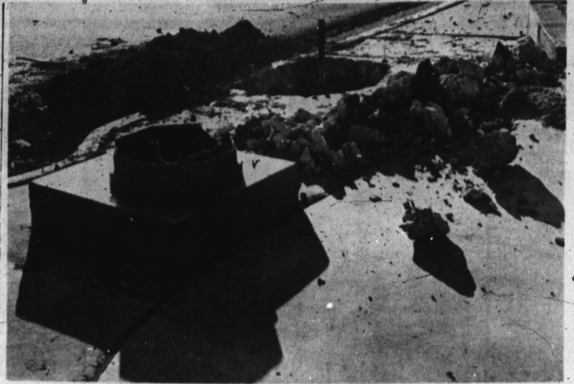
HEAVY DAMAGES — A Colorado truck causing extensive damages. (Hereford driver swung his trailer into a signal light Brand Photo) and fire hydrant at Park and Highway 385.
