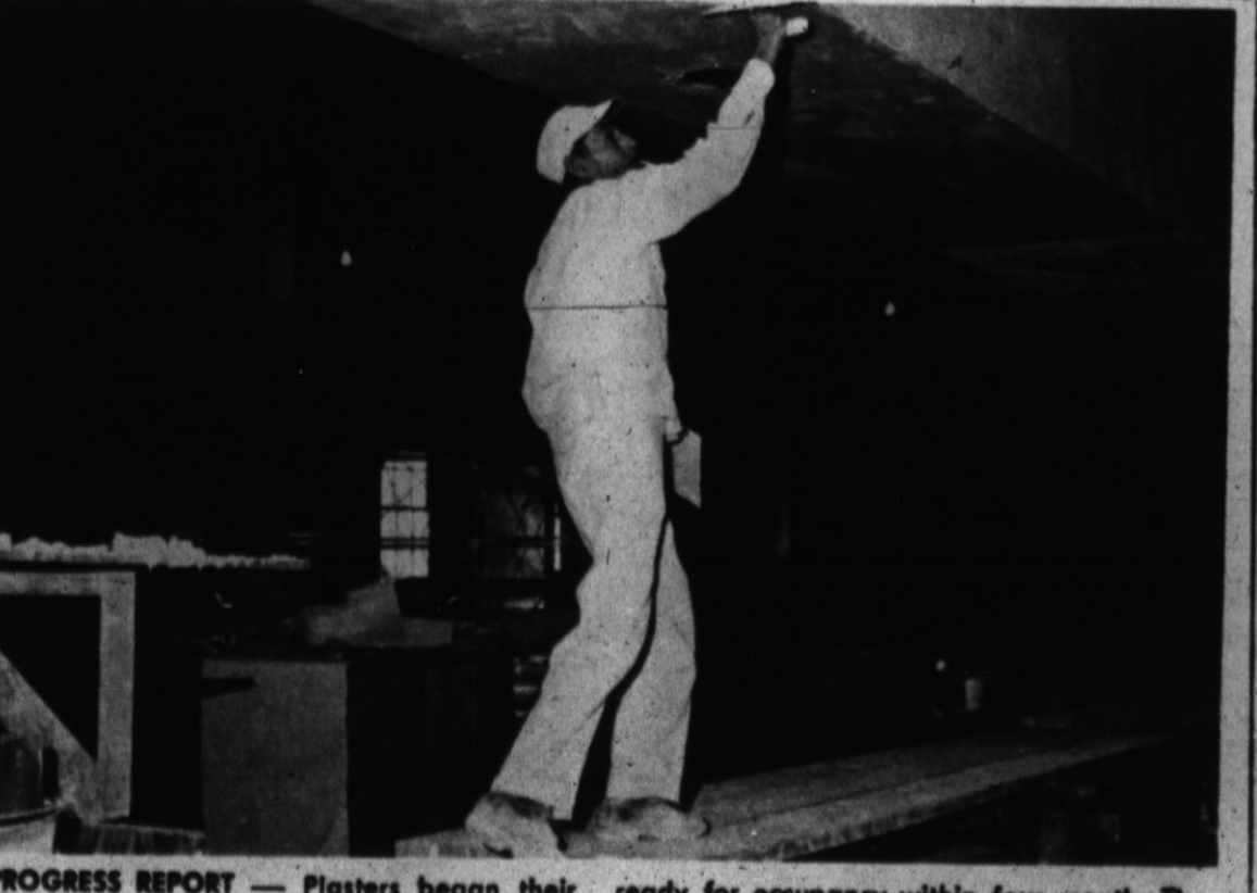
PROGRESS REPORT — Plasters began their work this week on the Post Office at Fourth and Main, where construction is 70 percent complete. The building is expected to be ready for occupancy within four month. The postal business is continuing at 313 Main. (Hereford Brand Photo)
