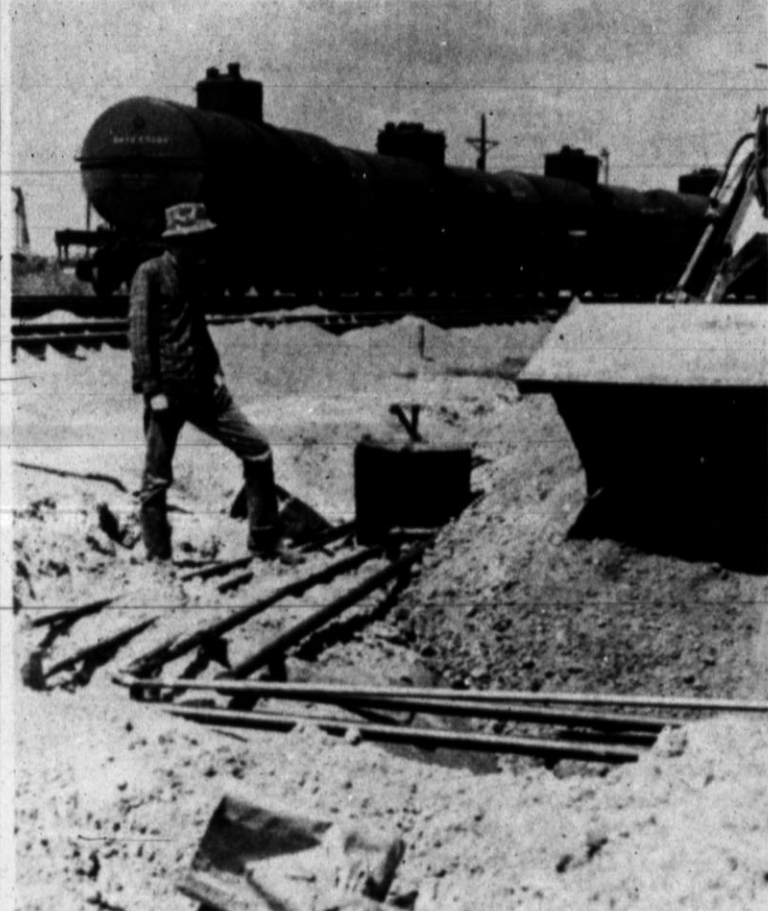
NEW BUSINESS ADDITION — Two 25,000 gallon underground storage tanks are being covered at the construction site of Pacific Molasses Co. as railroad tank cars stand by to take the first load. Unofficially, the thru-put station will begin operation Wednesday.
