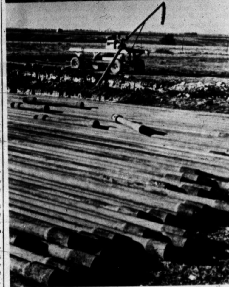
SALT MINE CONSTRUCTION — Work at the Hereford Salt Mines Inc., located about 5 miles south-east of Hereford on the Frio Draw has gotten a good start and is expected to be complete by early 1968. The salt will be mined by pumping fresh water into a 200-foot hole and subsequently dehydrate the salt in large tank type basins. The salt will be used as an ingredient for cattle feed.
