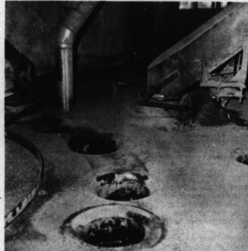
ON TOP OF the tall structures of Hereford Grain Corp. is the distributing section. The photo on the left shows where the grain is fed to each hole. From there, it goes to a
