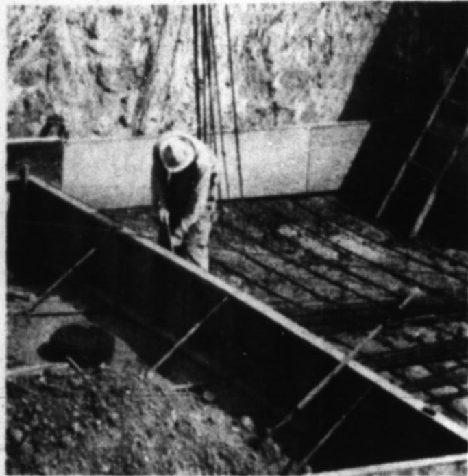
Allied Chemical Company . . . getting started on Progressive Road.
