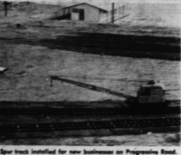
Spur track installed for new businesses on Progressive Road.
