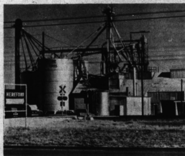
FAMILIAR SIGHT — Motorists going east on U.S. Highway 60 can't help but notice Hereford Feed Yards located just south of the tracks. The plant is six years old but still serves the need of the operation. (Hereford Brand Photo)
