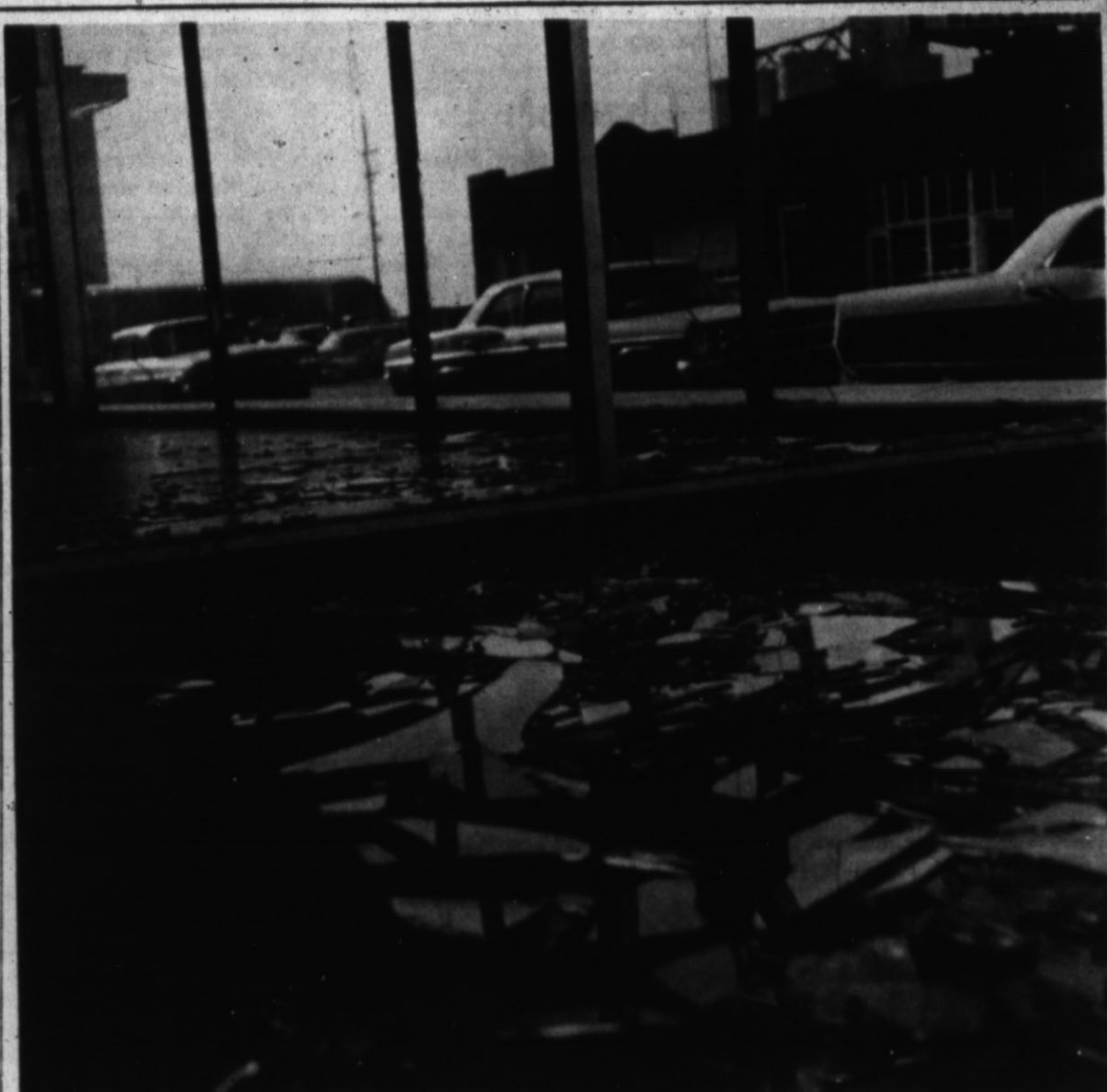
WIND DAMAGE — Kinsey-Osborn lost this day's wind. (Hereford Brand Photo) corner of their glass showroom during Fri-
