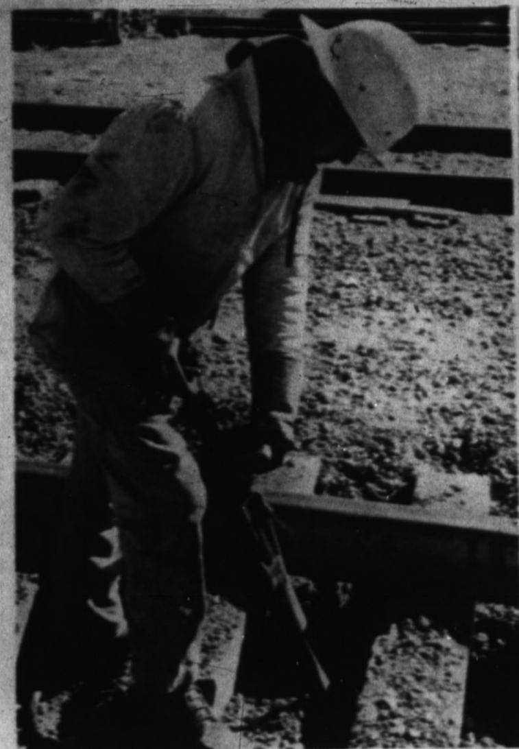
WINTER REPAIRS — Santa Fe crews were busy this week spreading ballast, putting in new cross ties and operating an automatic tamper. These men are using modern air
