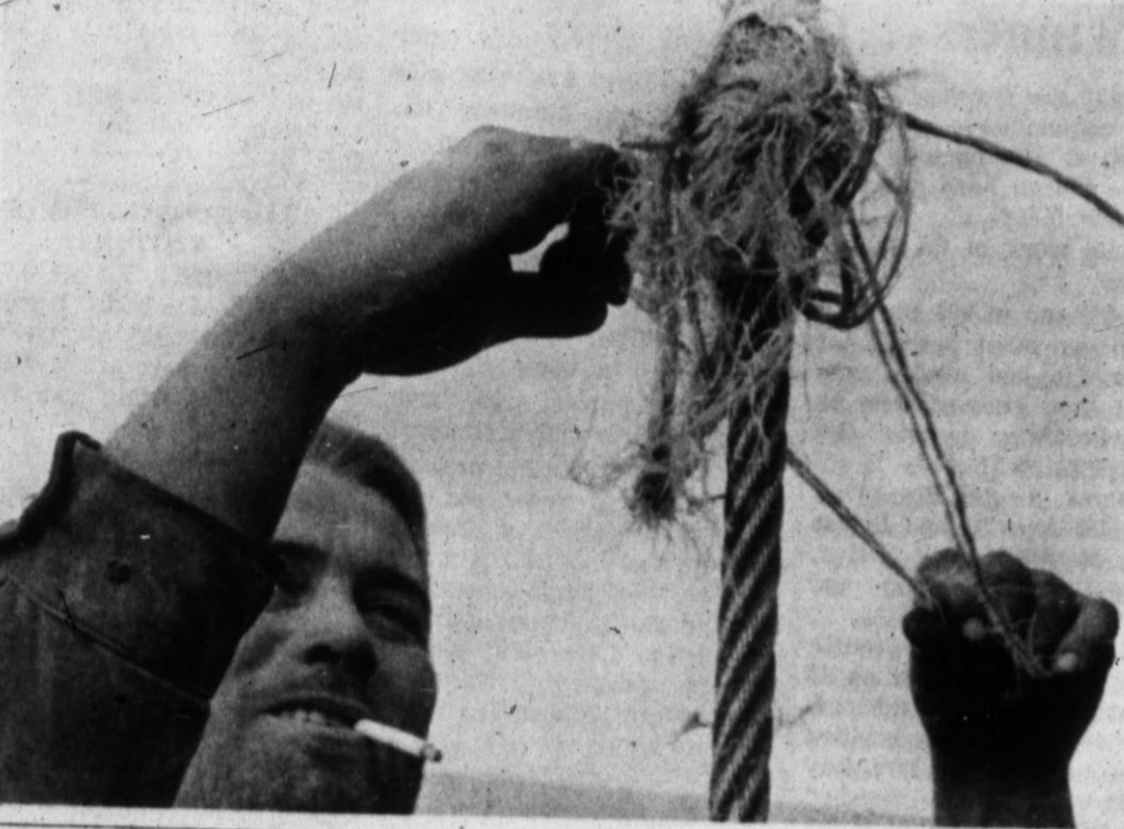
HOW FAR? Roughneck Roy Cassidy ties twine to the cable that lowers the bailing bucket into the hole. Water being taken from the well at this point cannot be tested because water is added to the hole as drilling progresses. After the hole has been bailed for several days, water can be tested. Hereford city officials are particularly watching for any signs of sodium chloride.
