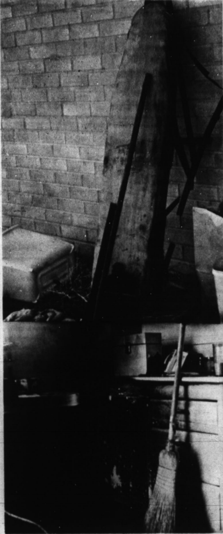
EFFECTS OF FIRES — A burnt ironing board, which had been placed beside a hot water heater, and a burnt cabinet, which had been the spot for cleaning a carburetor with gasoline, stand as mute reminders of the power of fire. See story in this issue for details. (Hereford Brand Photos)
