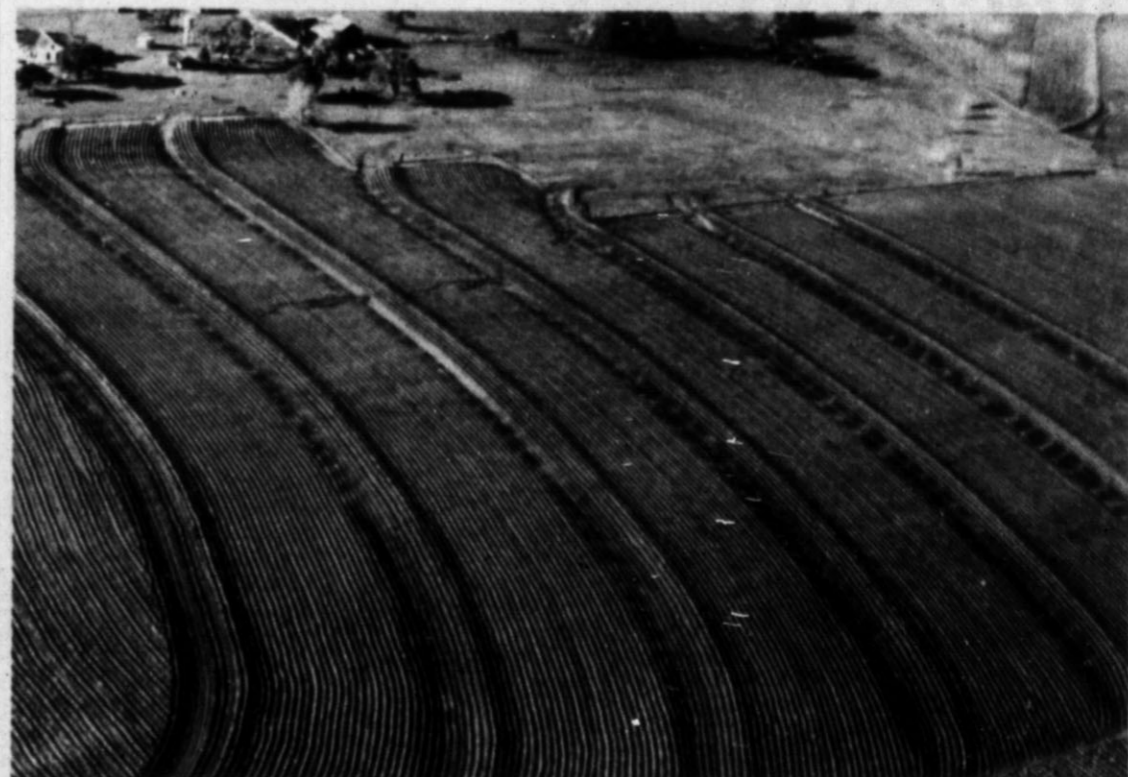
PATTERNS — This picture illustrates parallel terracing on a sloping farm. The slope is not steeper than the conservation practice is contraindicated. (Soil Conservation Photo)
