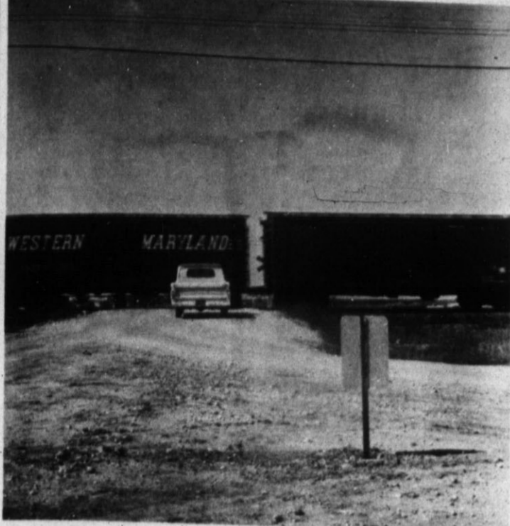
ACCESS ROADS — Hereford is being surrounded! New roads are circling the city. Shown is a recently completed railroad crossing two miles east of town. This makes a road cut through from Highway 60 to Dairy road useable. The
