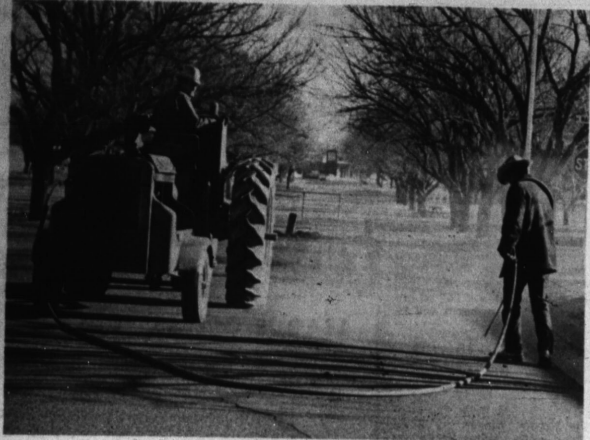
... clearing cracks of dirt with compressed air
