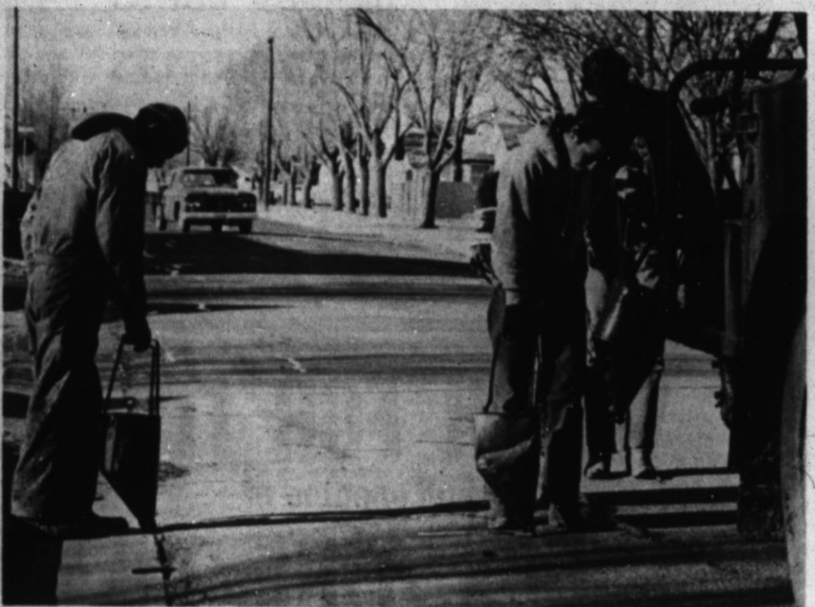
... hot tar is poured into cracks after they are cleaned
