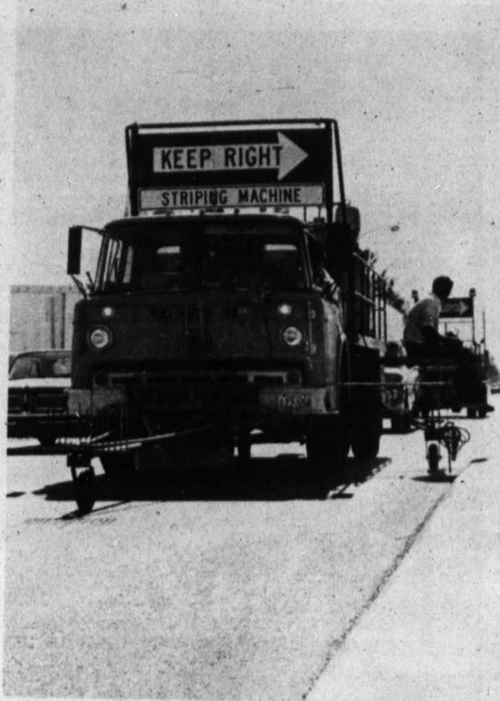
SIGN OF PROGRESS — Hereford streets took on an added sheen Monday and Tuesday as the Texas Highway Department crew painted in a number of new markers and added a fresh coat to old ones. (Hereford Brand Photo)
