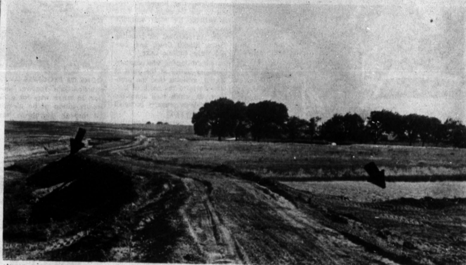
WHAT THE DAM DIVIDES — To the right of a dike constructed south of the Hereford Feed Yards is a horseshoe-shaped channel, used for the retention of possibly polluted water; the area is separated from the channel of the Tierra Blanca Creek, indicated by the arrow in the left of the picture. (Staff Photo)
