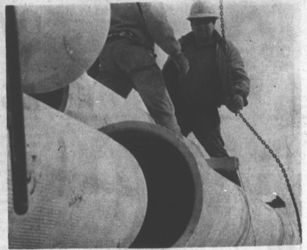
Through 12 inch concrete tile ducts . . .
