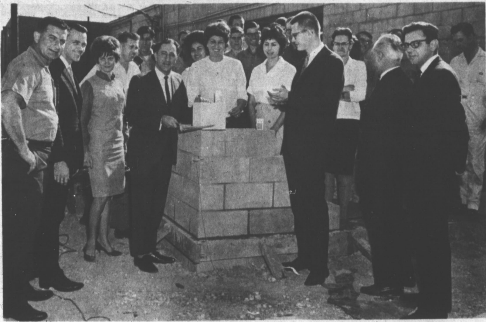
CORNERSTONE — Puzant C. Torigian, Bravo president, laid the cornerstone to the building addition at 1303 Park Avenue recently. Gary Daum, General Nutrition Corporation representative was on hand for the occasion. Other key personnel shown from left to right are Tony Ravizza, Company Engineer, Don Chapman - Hereford
