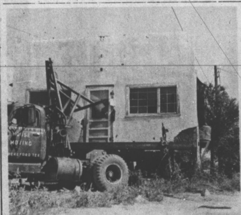
EYESORE BEING MOVED — A dilapidated building along 25 Mile Ave. and facing U.S. 385 was lifted from its foundation and toted away Saturday. The building was one of three recently declared as "unfit" by the city building inspector. (Hereford Brand Photo)
