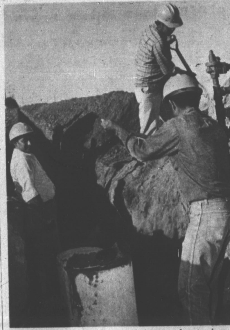
CONSERVATION — Part of the wise use of water is prevention of evaporation and absorption before the water gets to the crop. A major phase of the communities agriculture is the installation of underground irrigation systems. Joe Ramirez, Joe Garcia and Alachio Cordero are shown installing pipe on the Ewald Berend farm six miles west and two miles north of Hereford. (Hereford Brand Photo)
