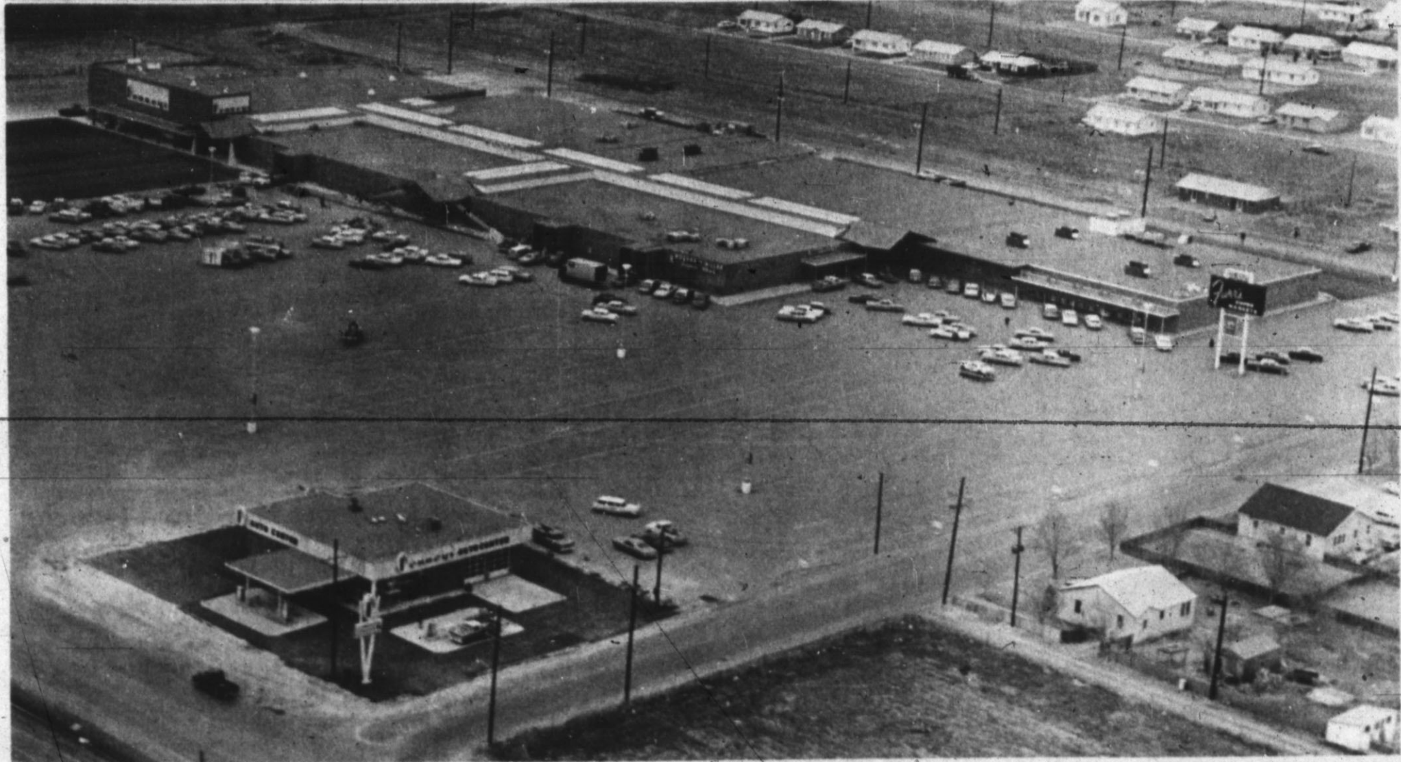
ECONOMY BOOSTER — Sugarland Mall Shopping Center — all 16 acres of it — marks the official opening of seven stores with a ribbon-cutting ceremony at 8:45 a.m. Wednesday. The north Hereford complex, viewed from a low-flying plane in photo above, is expected to help draw trade from throughout the Magic Triangle to Hereford, as described in story at right and in an editorial on page 6, section 2. (Staff Photo)
