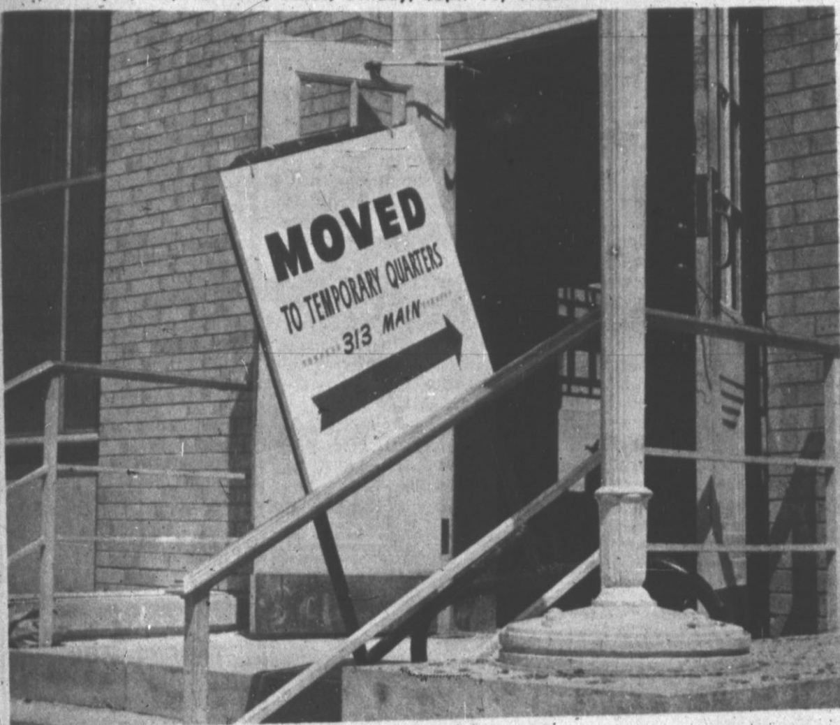
GO WHICH WAY? — Caught in the confusion of remodeling, this sign, intended to direct postal patrons to the temporary office building on Main has been ripped out. (Staff Photo)
