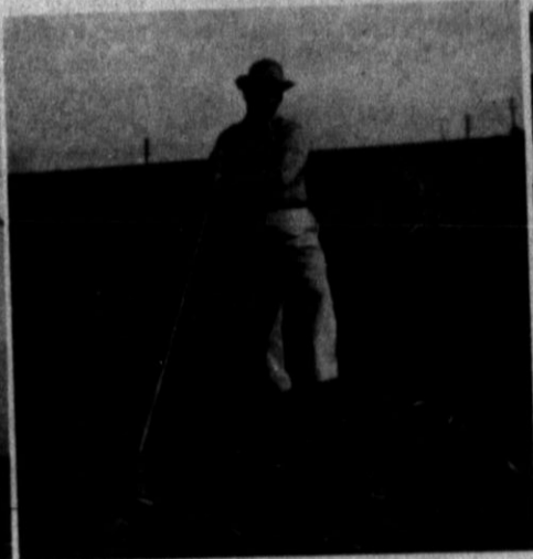
Marshall Formby digging foundation for KPAN building
