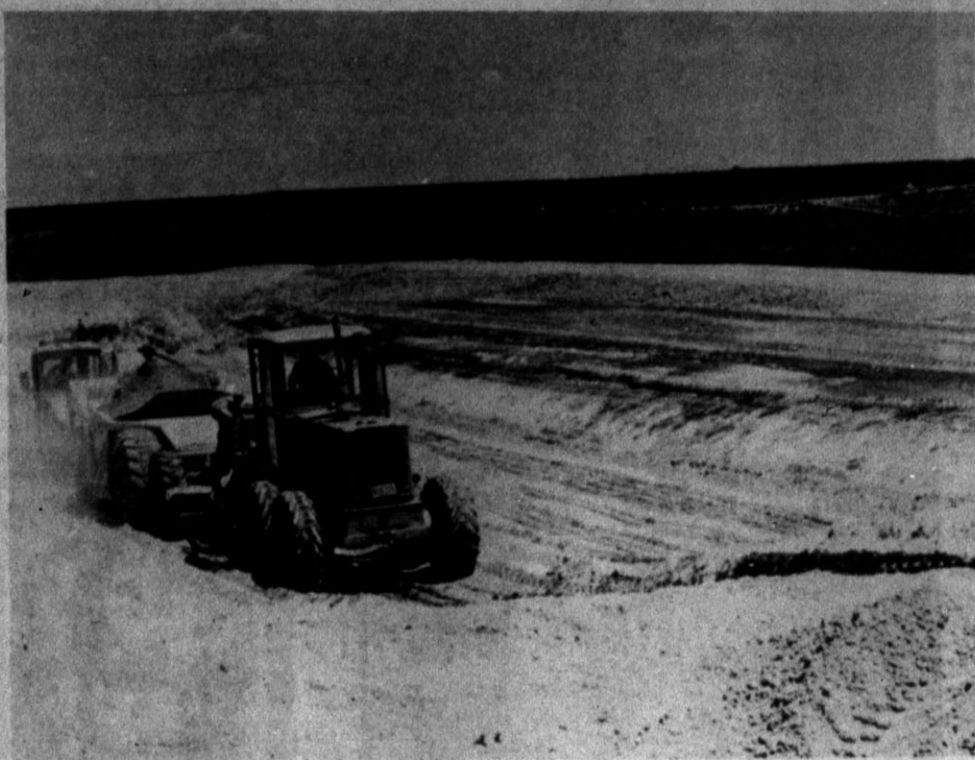
Clearing Dirt For Pond
