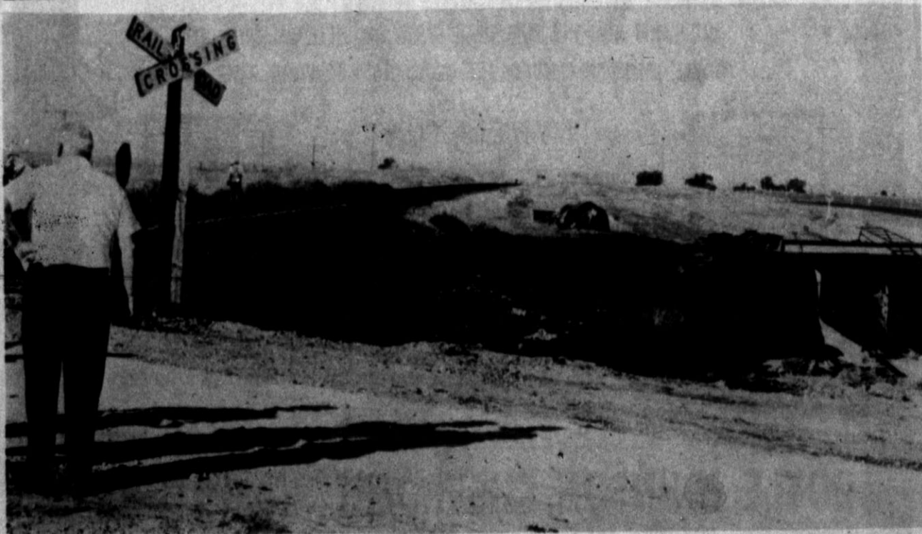
Hot Asphalt Spills Everywhere
