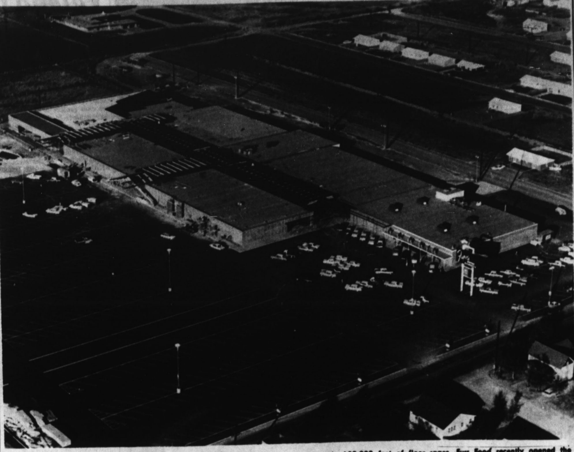
COMPLETION NEARS ON MALL —Construction of the Sugarland Mall on north 25 Mile Ave. nears completion as the final touches are put on the roof. The new mall will be completely air conditioned and will cover approximately 120,000 feet of floor space. Furr Food recently opened the first store in the mall. (Staff Photo by David Butler)
