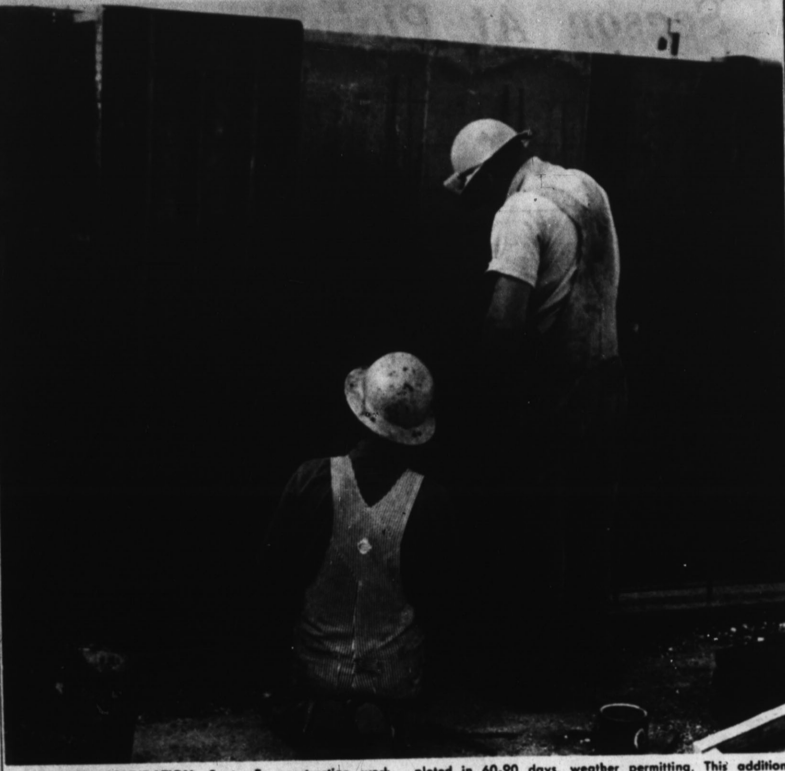
COMPLETES FOUNDATION —Santa Fe construction workers finish setting up the metal forms so that the cement foundation can be completed on the addition to the Santa Fe Depot on Hwy. 60. The addition is expected to be completed in 60-90 days, weather permitting. This addition will be used for rail and truck freight storage at the depot. (Staff Photo)
