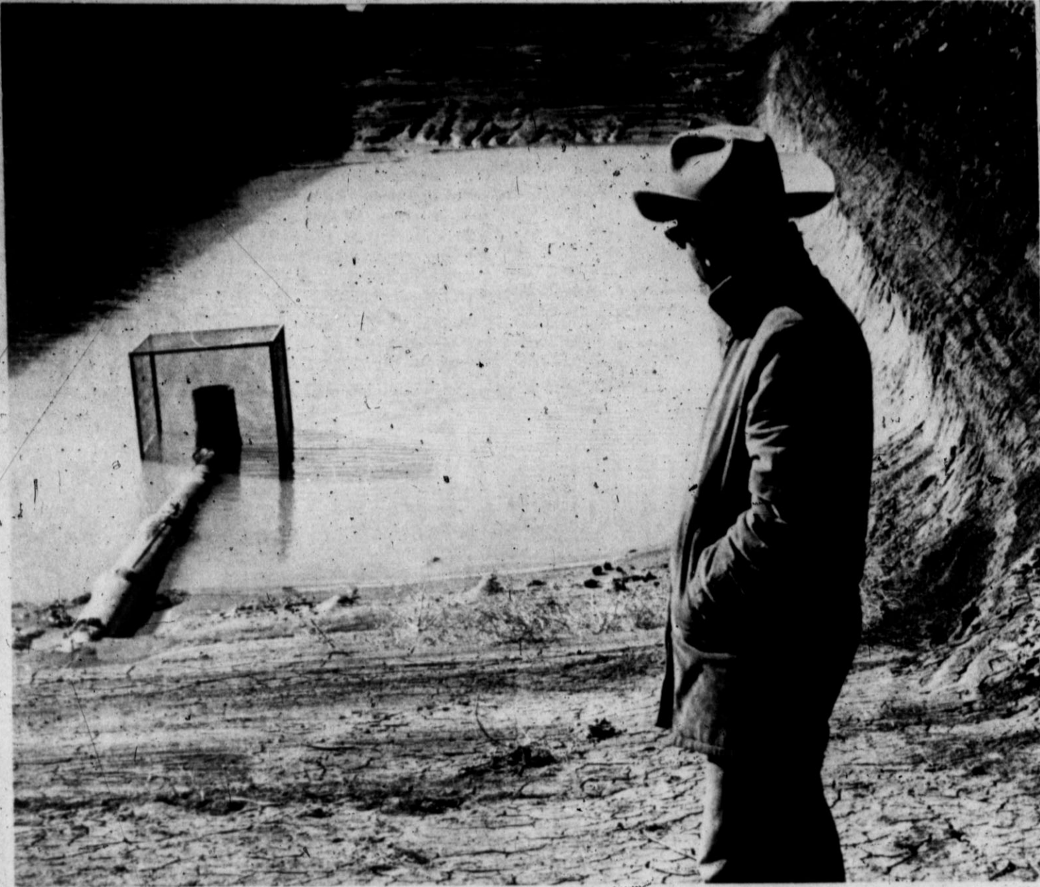
AN INSIDE VIEW — is what local farmer Jim Thomas is getting of this tailwater pit recovery system. It is only one of many installed in Deaf
