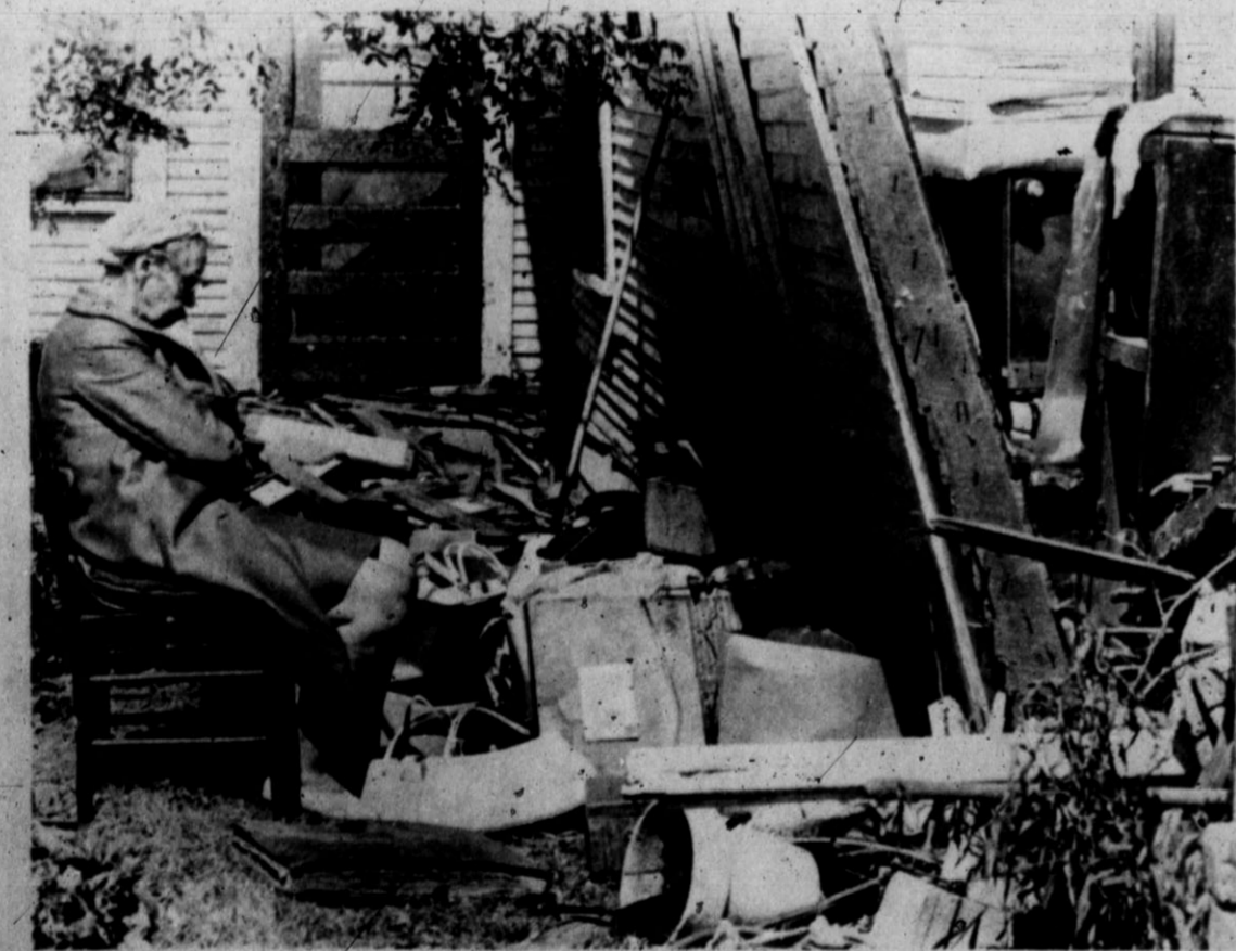
WIPED OUT — Mrs. Ruth Thomas, 76, of Lubbock, survived the tornado which tore through the heart of the city by hiding in the closet of her home, almost the only part of the structure left undamaged. Here, sur-
