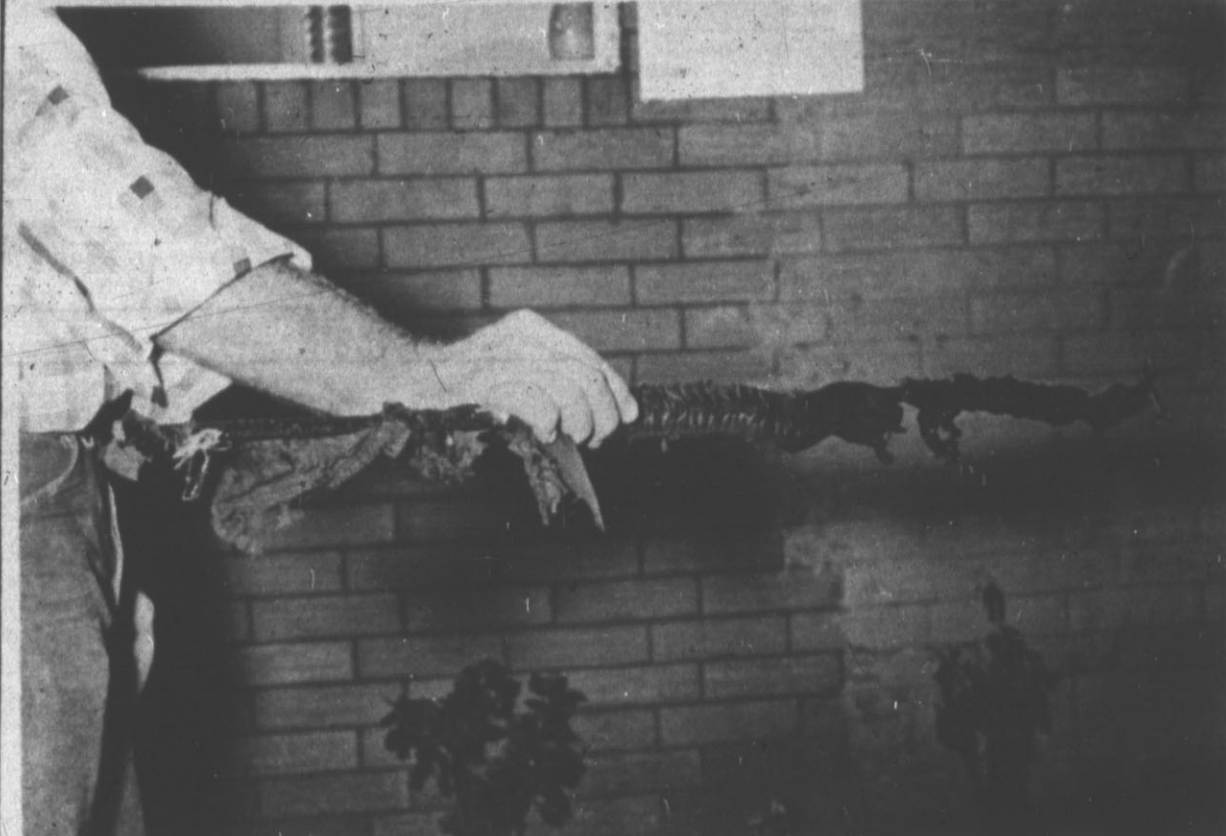
MINOR DAMAGE — Damage to bathroom. The fire was caused by a heater under the curtains resulted from a fire at the home of the curtains in the bathroom. (Hereford Brand Jim McDowell, 205 Emma, Friday afternoon. Photo)
